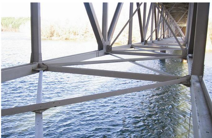
Figure 5. Lower lateral bracing system on truss bridge
