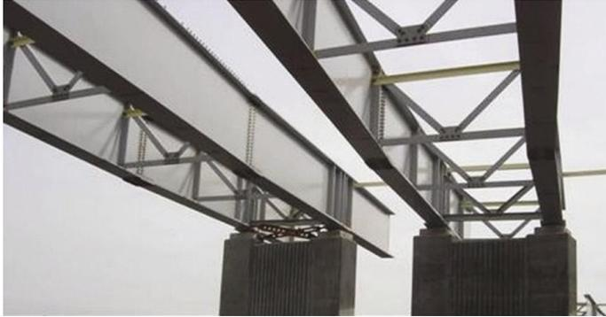
Figure 1. A pair of braced steel beams.
