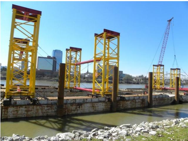
The arch support on falsework is modeled to realistically limit the transfer of lateral force to the falsework as a function of the vertical load present with a "frictional contact" joint material.
