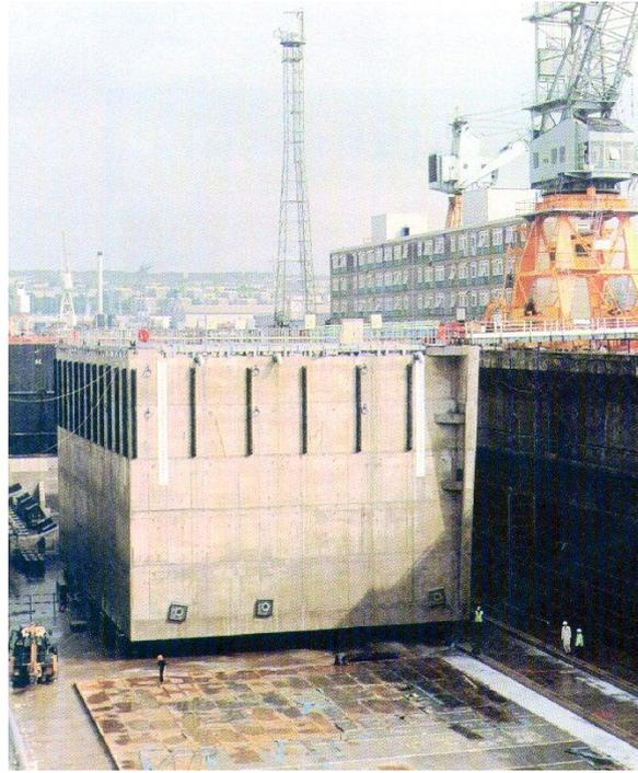
**Fig. 9– Dock caisson under construction**
