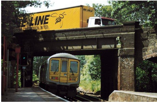
Figure 3. Over-bridge at Hackbridge, UK.
