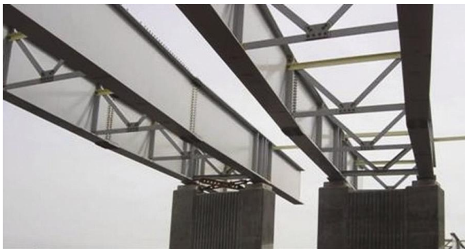
Figure 9. A pair of braced beams.
